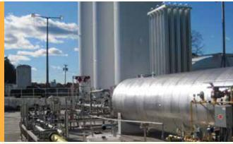
Chart provided a complete turnkey solution to provide LNG as the source for combined heat and power (CHP) at a remote diamond mine located in Quebec Canada and completely off both the electric and natural gas grids.
