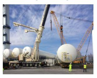
Four million litres of liquid nitrogen and oxygen storage being installed at an industrial gas facility in Finland.
