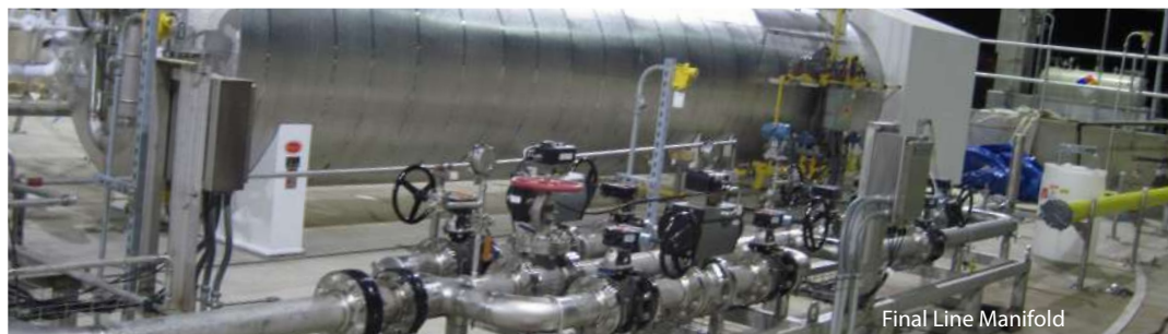
3 tanks, vaporizer, IFWB and manifolds
